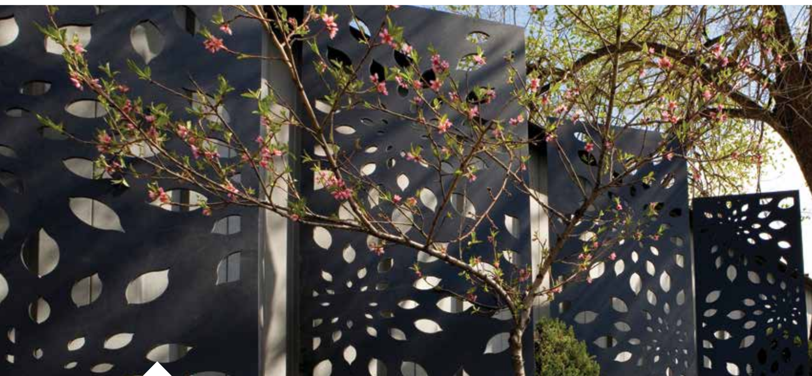
Pattern: Lemon Drop [ contemporary ] Project: Larea Residence (Mexico City) Material: 1/4" aluminum Support: 48" on-center
